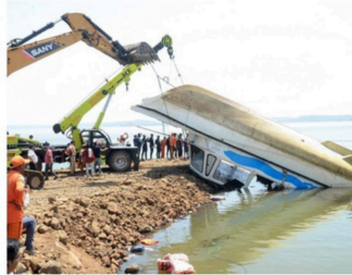
Officials recover the cruise boat, which overturned in the Bargi Dam due to a sudden storm, from the Narmada river in Jabalpur. ANI
