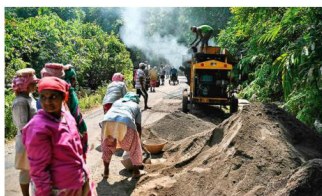
Construction workers build a road cutting through forest land, as part of the Great Nicobar Island Project. AFP
