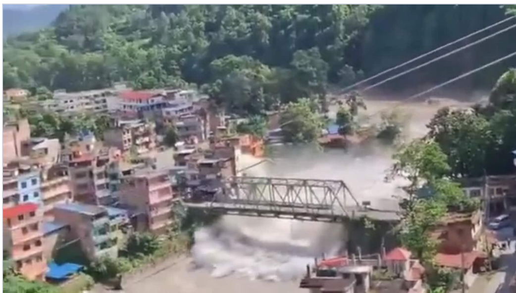
Flood fury: A truss bridge is overwhelmed as the debris flow tears through a hillside settlement near the Nepal–Tibet border.
